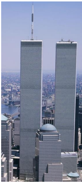
The Twin Towers with the Communications Tower atop the North Tower Image: Public domain
